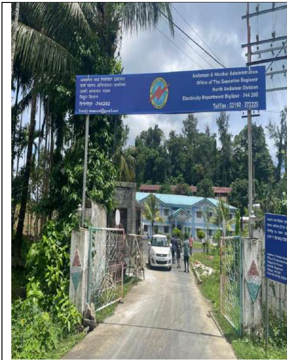
Office of the Executive Engineer
