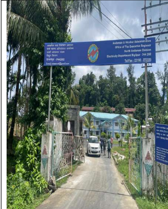
Office of the Executive Engineer
